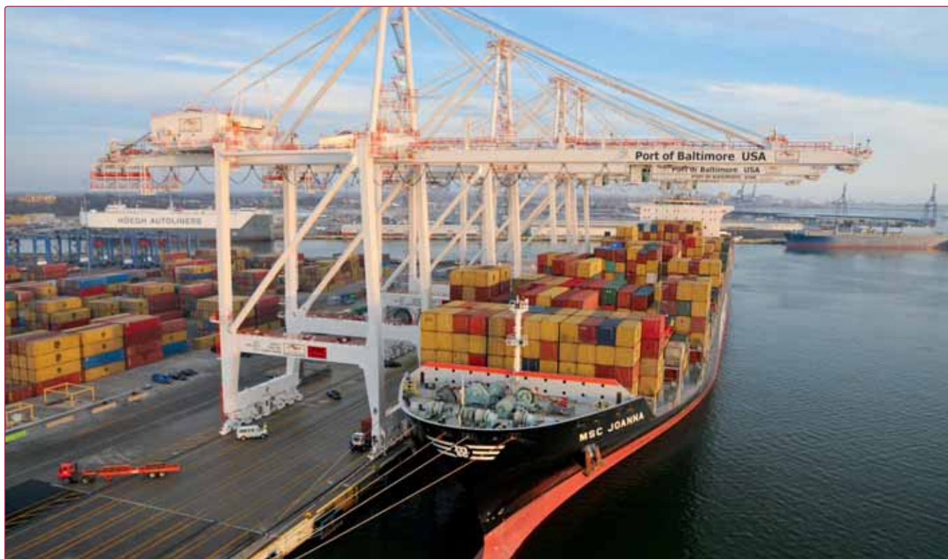
Ports America Chesapeake's Seagirt Marine Terminal, Baltimore, Maryland, USA
