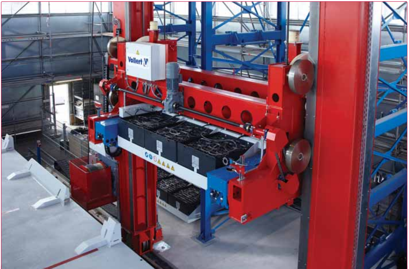
Figure 3. Fully automated battery-changing station.
