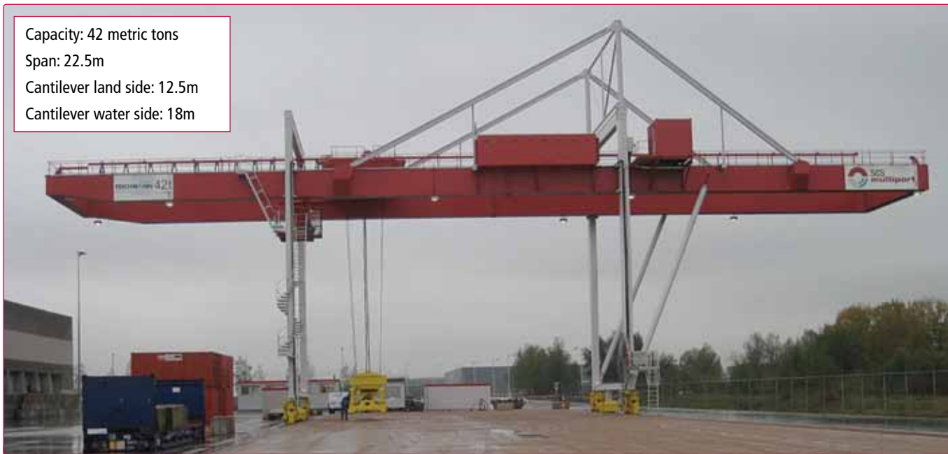
Container crane after reconstruction.
