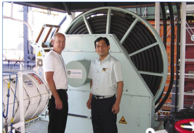
Figure 1. Electrical cable reel on ship.
