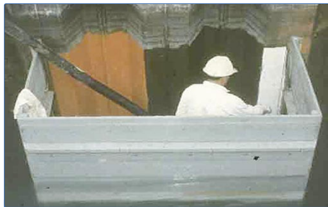
Applying coating from cofferdam to quay wall of steel sheet piling.
