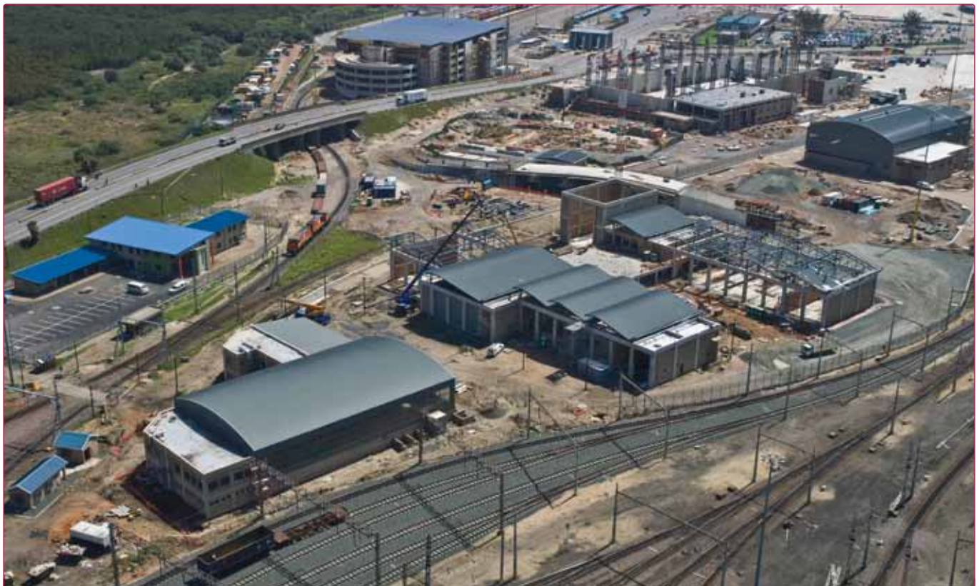
Durban container terminal's R1.4 billion capacity creation project includes the relocation of workshops and infrastructure away from the quayside to create additional container stacking area.
