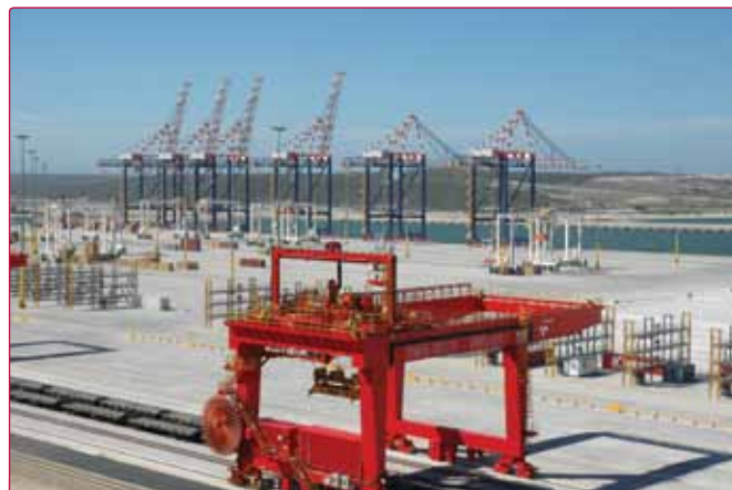
Ngqura container terminal's rail-mounted gantry cranes with Liebherr ship-to-shore cranes in the background.
