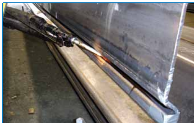
Figure 2. Wadit can be quickly and efficiently applied into any steel sheet piling interlock including cold formed sheets like that above.
