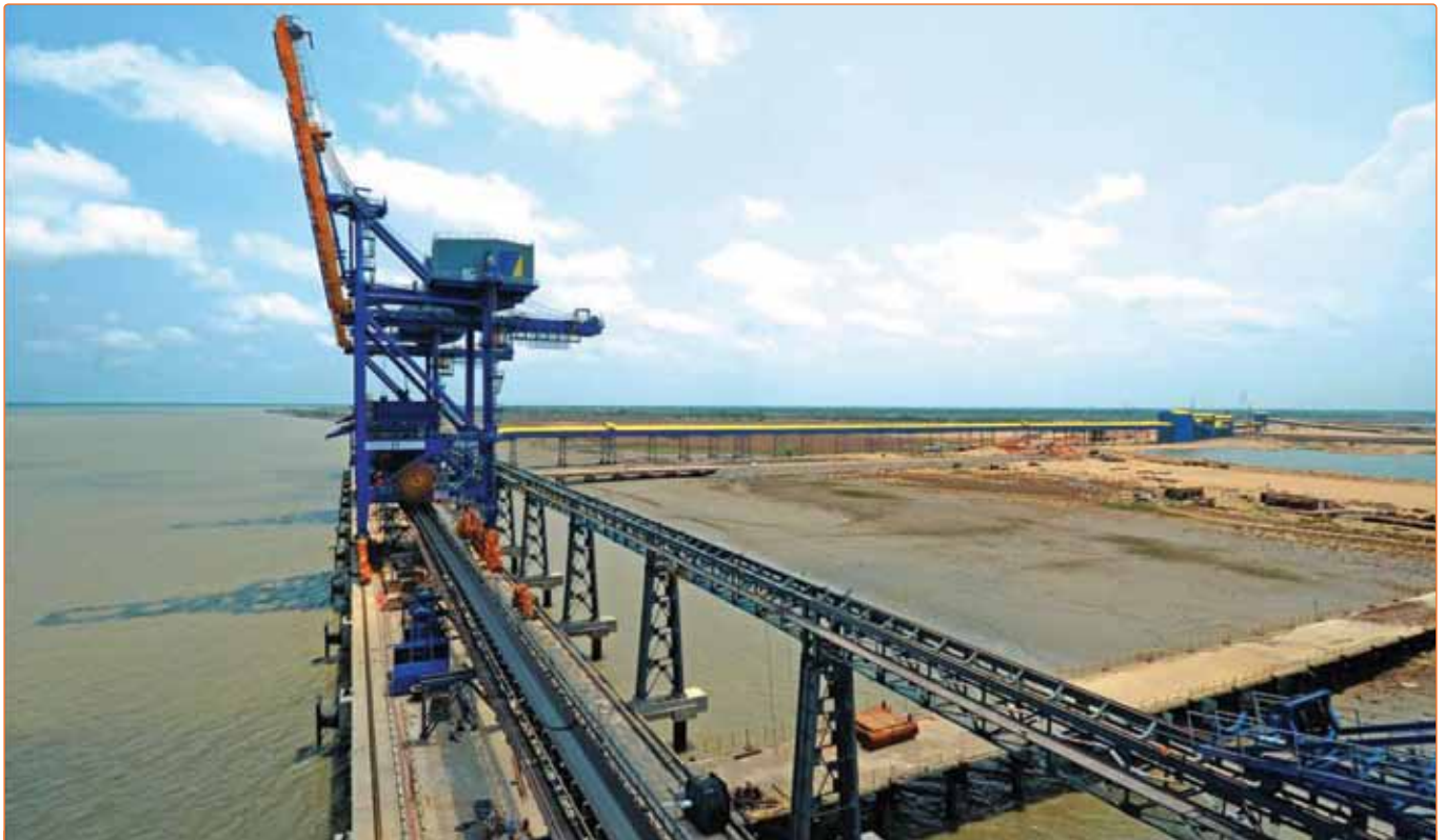
Overall view of the jetty with its approach.
