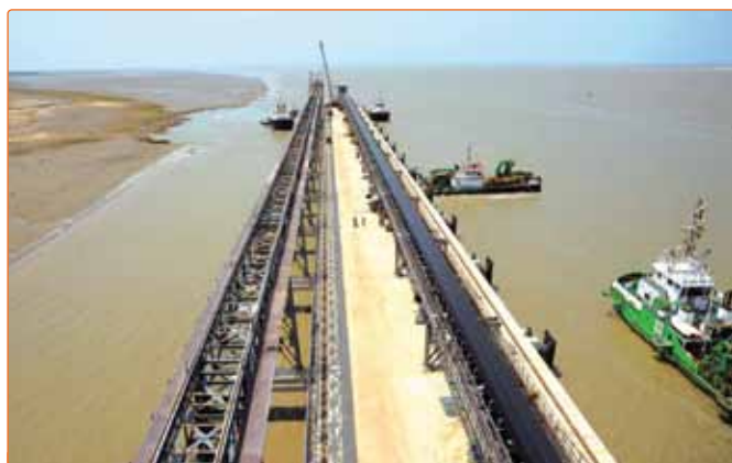
Top view of the jetty with its conveyors.
