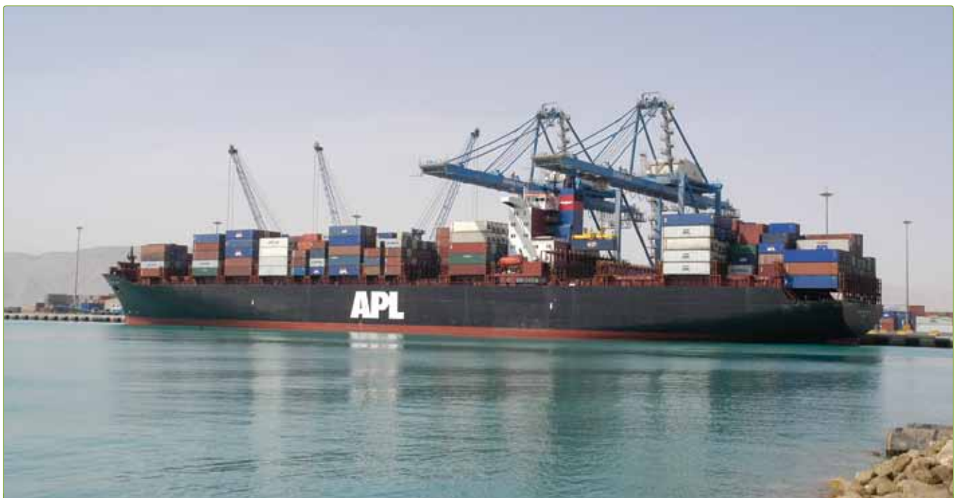
DP World-Sokhna is perfectly positioned to handle cargo flows of up to several million tons and 750,000 TEU containers per year into and out of Egypt and the wider Middle East region.
